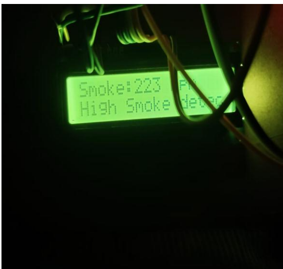
Figure 1b. High smoke detected and displayed in LCD display.
