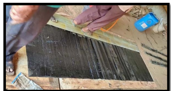
Stick Bamboo sheet on Bitumen sheet
