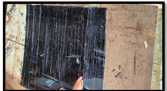
Bitumen Sheet to stick Bamboo sheet
