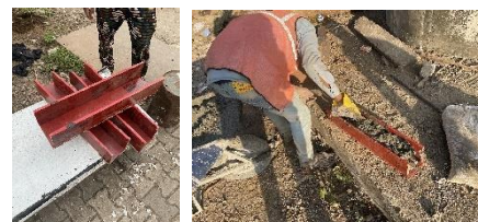
Fig -2: Wooden Concrete beam molds and Casting of Specimens.
