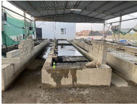
Fig -3: Curing in special saline tanks.
