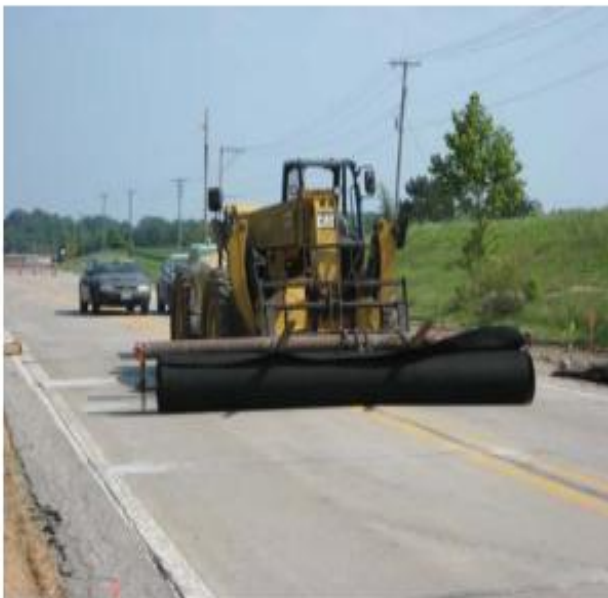
Figure 7 – Geotextile Fabric Placement
