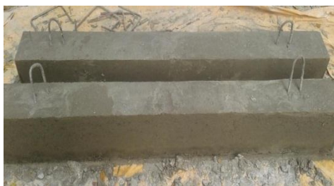
Figure 1 Casting of RC beam specimen.
