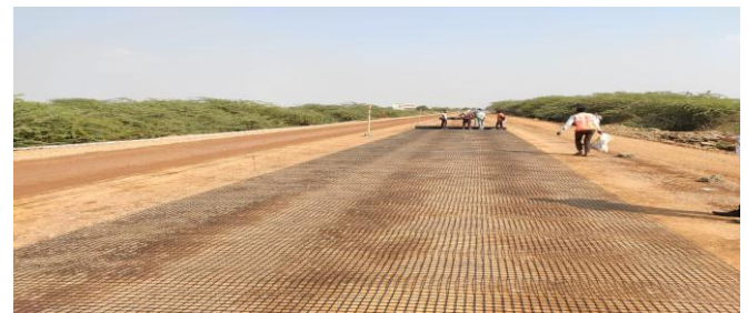
Fig -1: Laying Geogrid at Site
