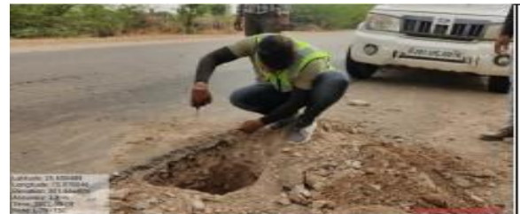
Fig -4: Trial Pit of Existing Pavement
