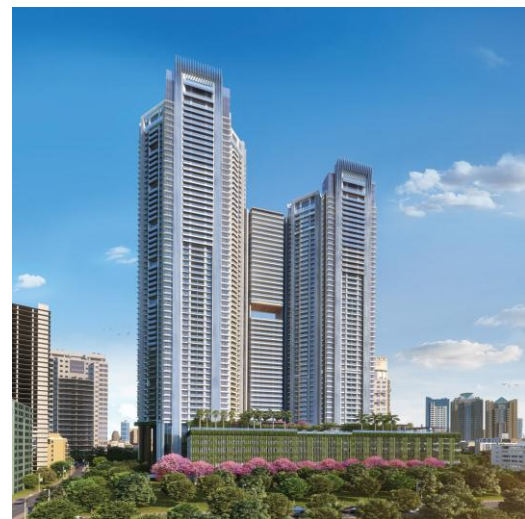
Fig -1 Resting on A Flat Ground
