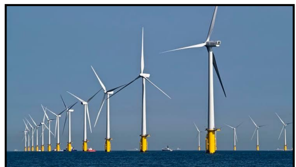
(Fig:-1.3 Off-shore type of wind turbine)
