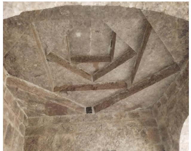
Fig -9: sandstone masonry square stepped slab
