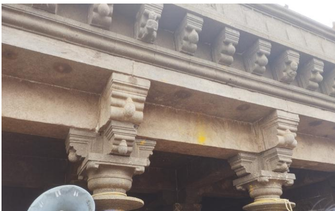
Fig -5: sandstone beam and slab of main temple
