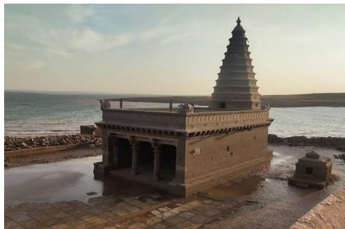
Fig -12: Basalt stone used in main temple structure
