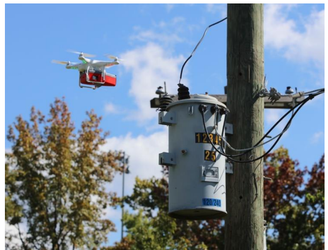
Figure 5. Drone inspecting a distribution transformer.
