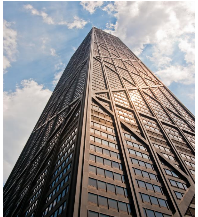
Figure 1 John Hancock Center in Chicago, example of the trussed tube structural design
