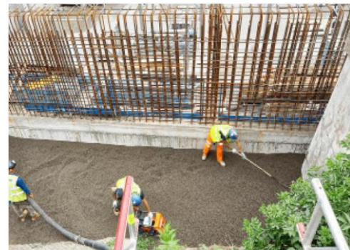
Fig. - 6: LECA LWA Fill behind Retaining Wall, Bristol [3]
