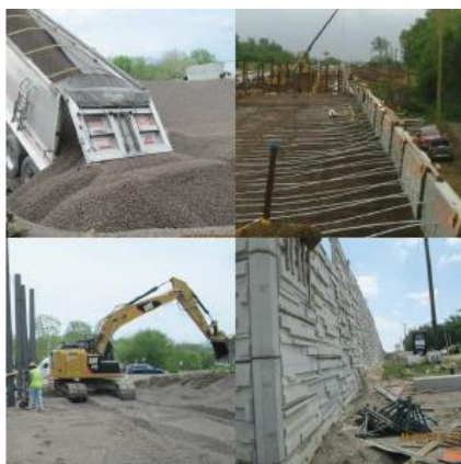
Fig. - 5: ESCS LWA Backfill behind MSE Walls, Indiana [2]
