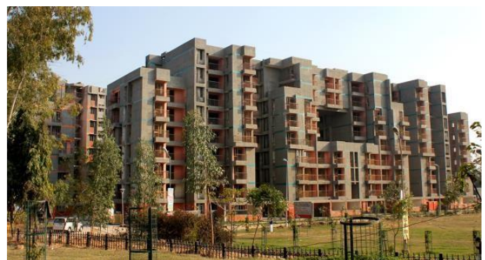
Fig -8: View of Mega Housing project Plan [12]
