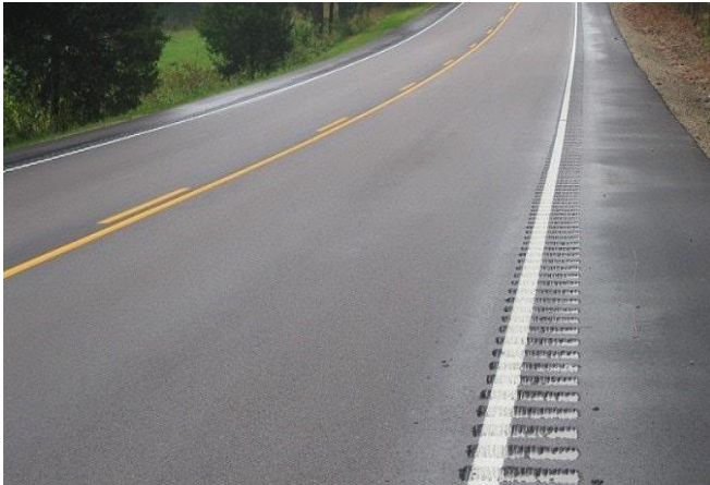
Figure-02: Flexible Pavement
