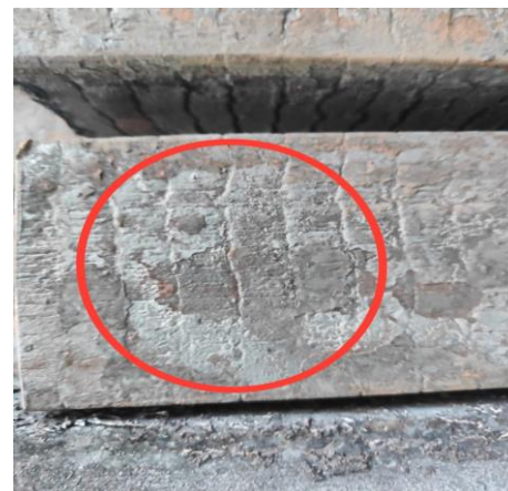
Fig 6: Transverse Crack
