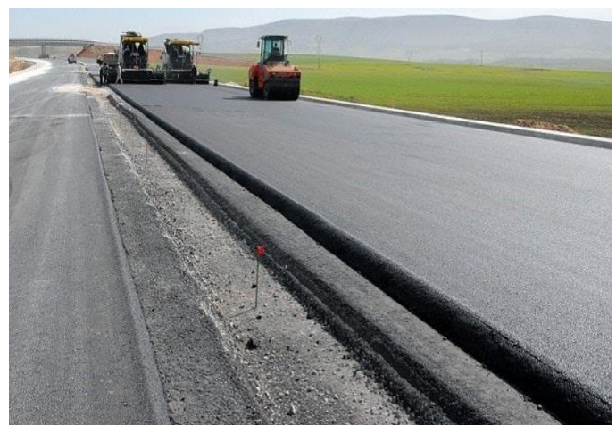
Figure-1: Highway Pavement
