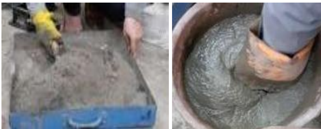
Figure 2 Mixing concrete.
