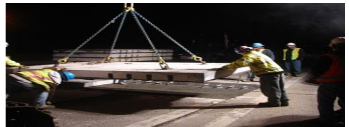
Fig.1.8: Reusable Road Panels.
