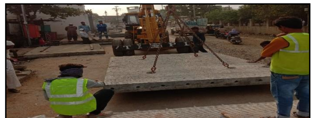
Fig.1.4: Placing of Panels.
