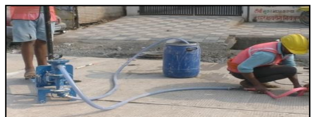
Fig.1.5: Grouting of Panels
