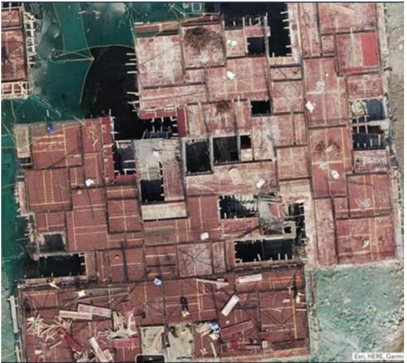
Fig -3: Image shows Tower 1 Slab Shuttering and Reinforcement work in Progress.
