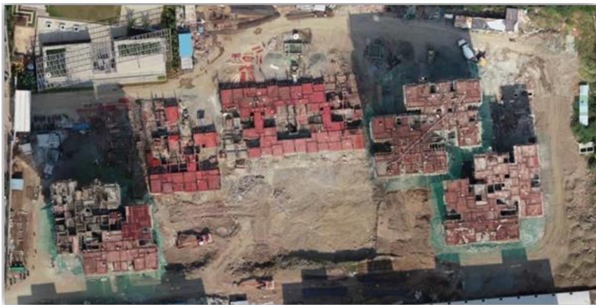
Fig -1: Raw Drone Capture of the Project including 5 Towers
