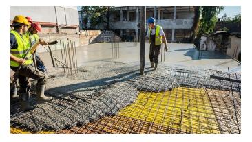
This concrete is made of cement, coarse gravel and water and steel or iron bars helps in reinforcing the materials mentioned before. The steel or bars get embedded in the concrete and it makes the construction super strong and durable.
