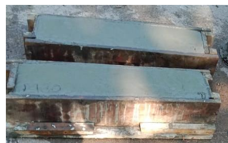
Fig-3: Casting of Beam
