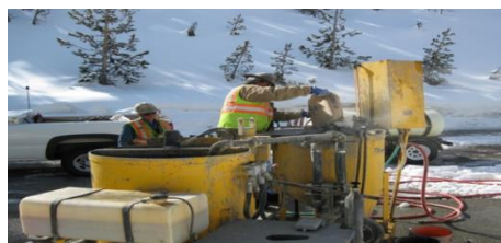
Fig3c: A typical grouting facility. Picture provided by Barry Siel, FHWA. (Carlos A.Lazarte, 2015)
