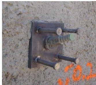
Fig3a: Solid tendon in a photograph that has a steel plate, a washer, and nut studs that are not headed for attachment to the final facing. Thanks to DYWIDAG-System International for the image. (Carlos A.Lazarte, 2015)
