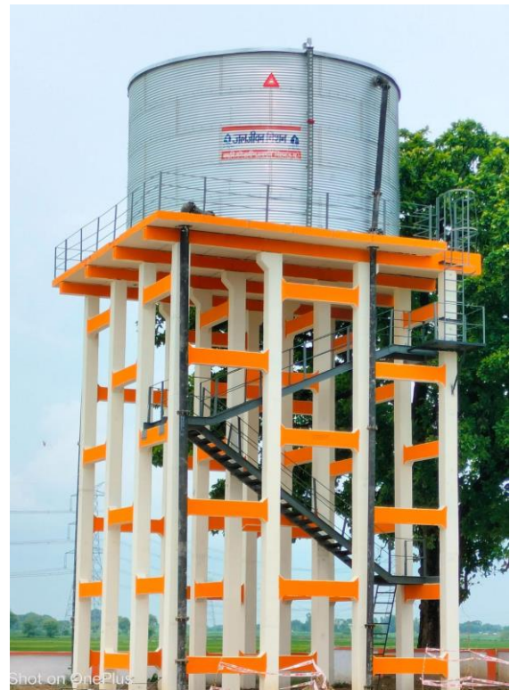
Fig -1: Precast Water Tank
