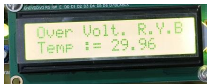
Fig.10. over voltage fault detection on LCD display
