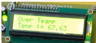
Fig.14. Over temperature fault detection on LCD display
