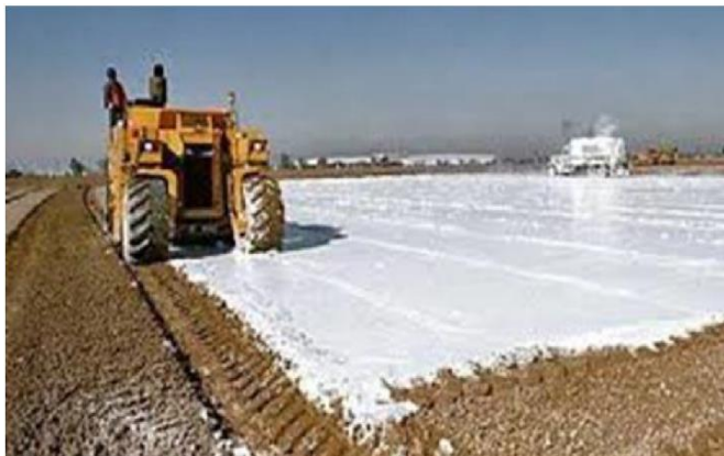
Figure-2: Lime Stabilization
