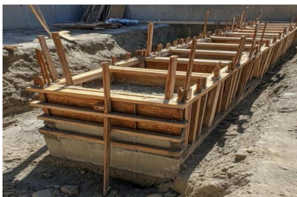
Fig 19 Conventional formworks
