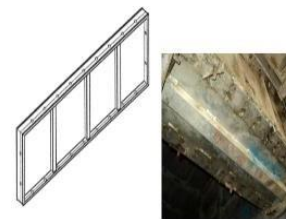
Fig 5 Beam Side Panel Beam Side Panel
