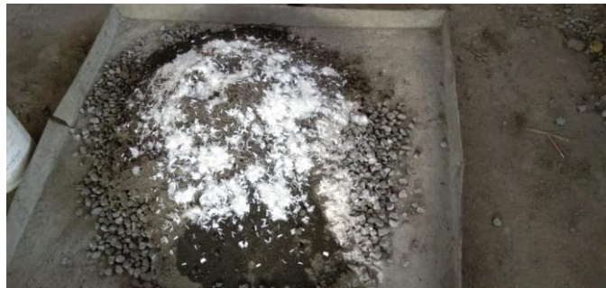
Figure 1 Casting of Concrete
