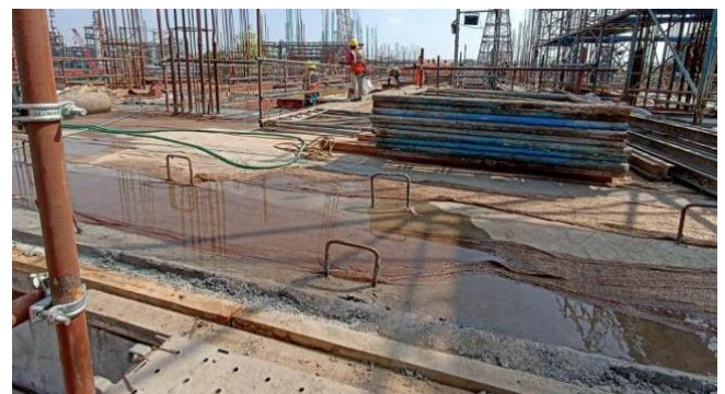
Fig. 12: Concreting the slab
