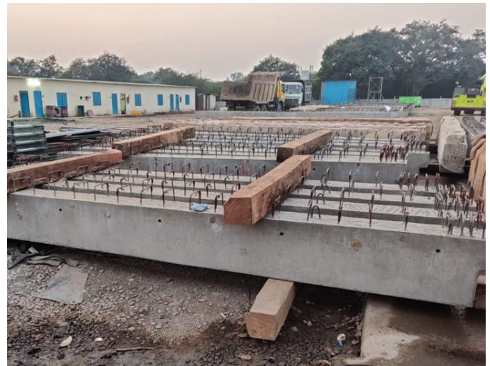
Fig. 6: Stacking of cast components
