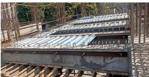
Fig. 10: Fixing ISMC channel & deck sheet
