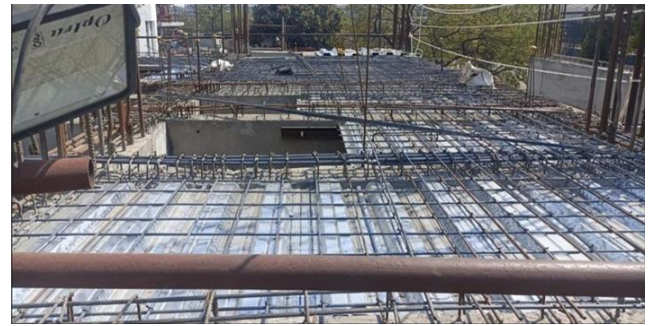
Fig. 11: Laying slab reinforcement
