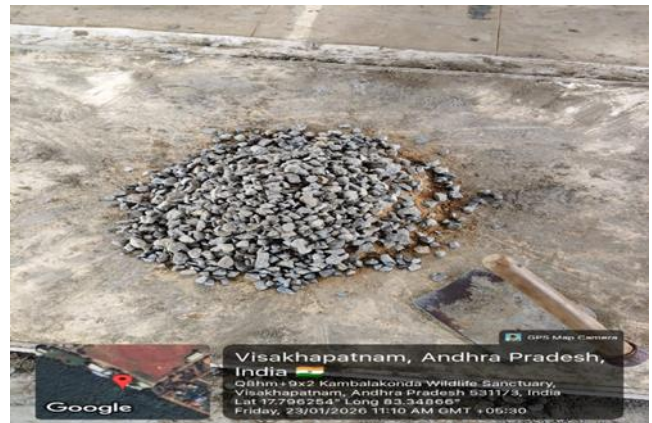
Fig :4 dry mixing
