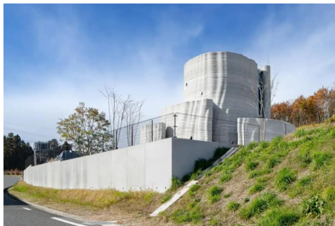
Fig 2: 3D printed earthquake resistant house developed in Japan
