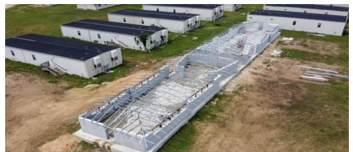
Fig 1: 3D printed military barracks developed using large scale concrete printing technology
