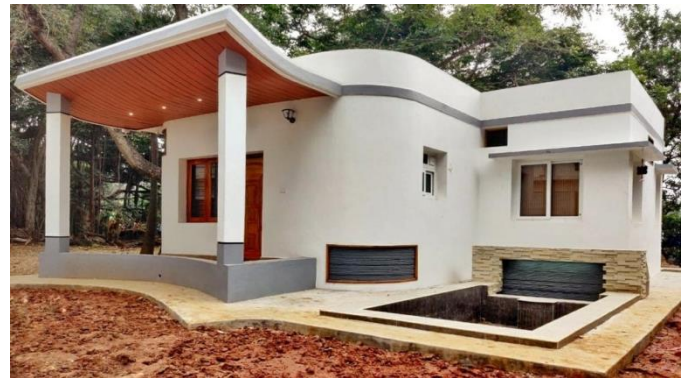
Fig 3: 3D printed house constructed by Tvasta at IIT Madras
