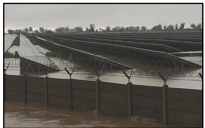
Fig -5: Flood Impact on Solar PV module
