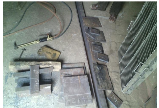
(Fig.4 Gas cutting setup)
