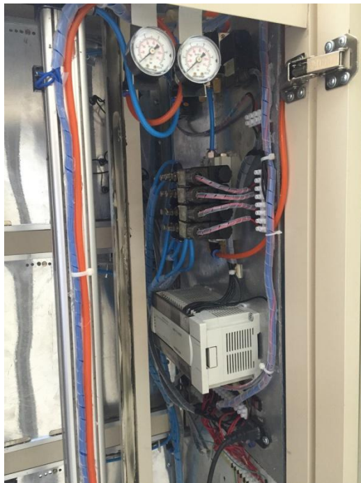
Fig-5: pneumatic and electrical circuit
