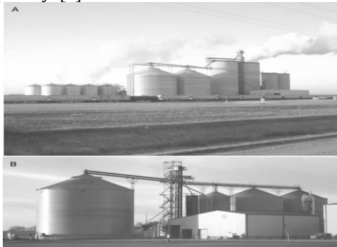
FIGURE 2. U.S. dry grind corn-to-ethanol manufacturing plants. A. 450 \times 10^6 L/y plant. B. 80 \times 10^6 L/y plant.
