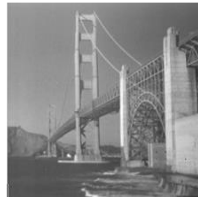
Figure 5. Original Bridge image
