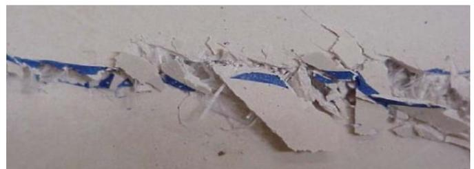
Fig.8: Longitudinal cracks
