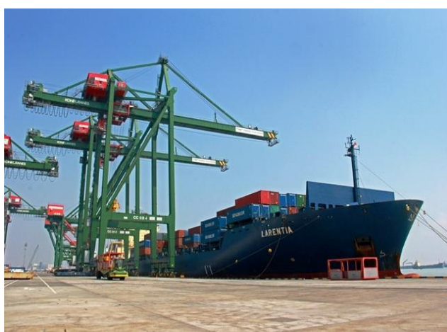
Fig -2: Ship to Shore (STS) Cranes
