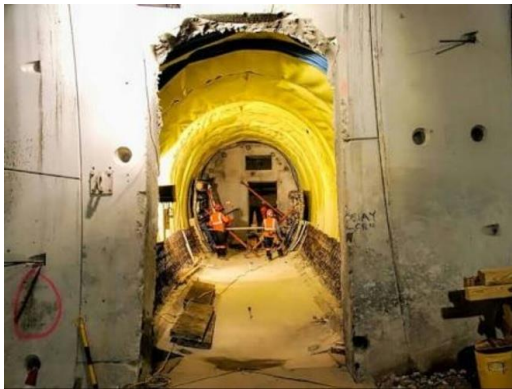
Fig.1: A Typical Horse Shoe Shaped Cross Passage
