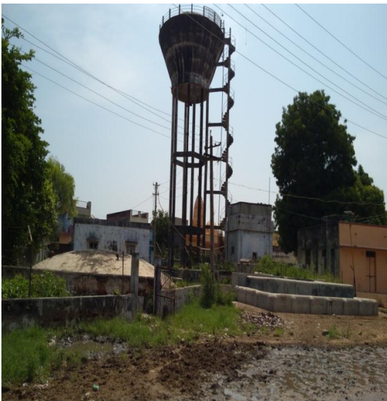
Fig 3:- Elevated storage Tank (1 lakh Litres)
