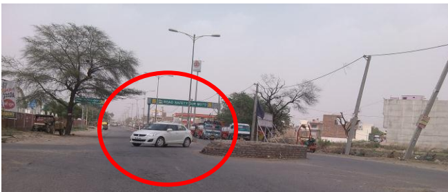
Fig. -5: Wrong crossing of vehicles around the rotary due to non-existence of traffic lights, traffic signs & symbols nearby Old bus stand, Barwala.
