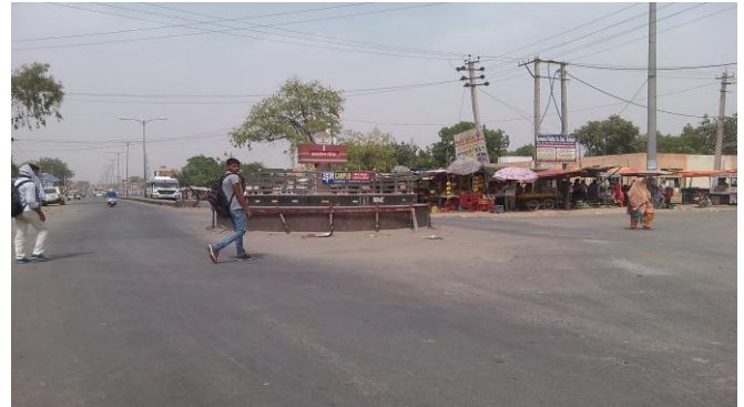
Fig. -7: No pavement markings for vehicles and pedestrians with unprotected 4-leg intersection. Delineators are in poor condition nearby Agrasen Chowk, Barwala Road.
