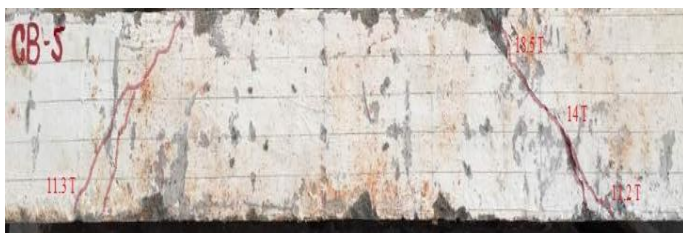
Crack pattern for control beam
