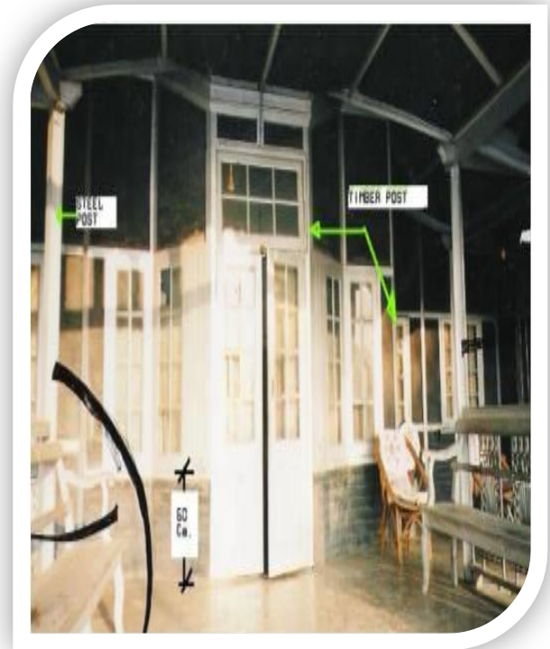
Fig -7: Ceiling and floor
