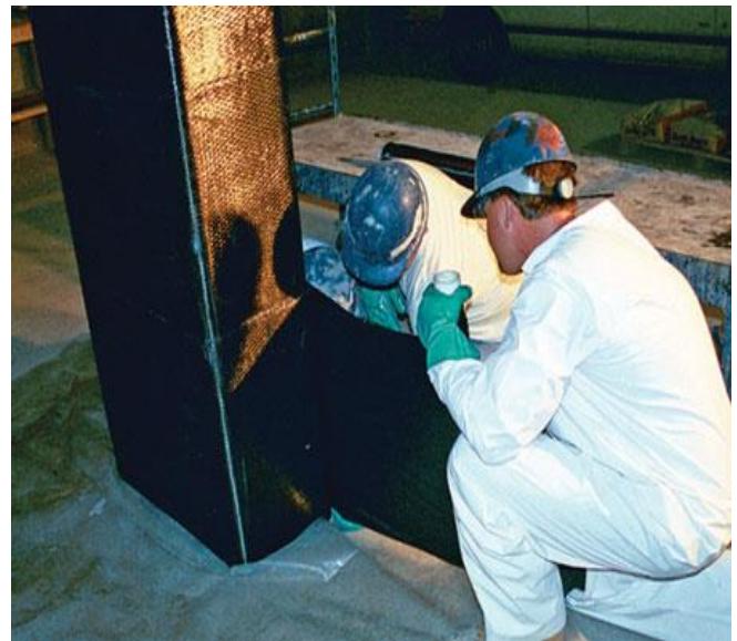
Fig -1. RCC column retrofitting
