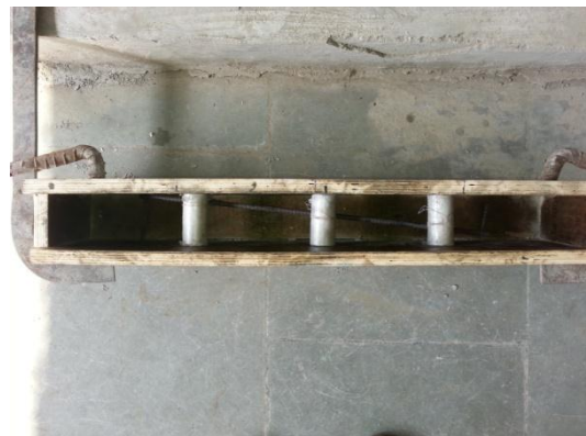
Fig. 4 Formwork prepared on site.
