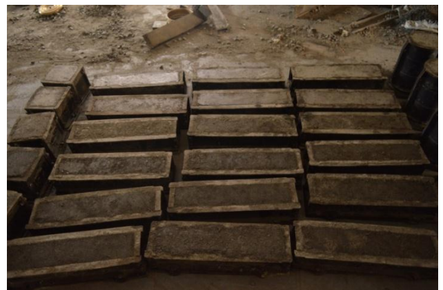
Fig -1 Moulds After Filling of Concrete
