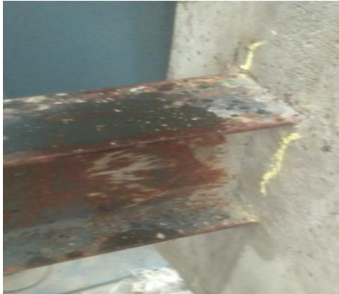
Fig 8 initial crack
