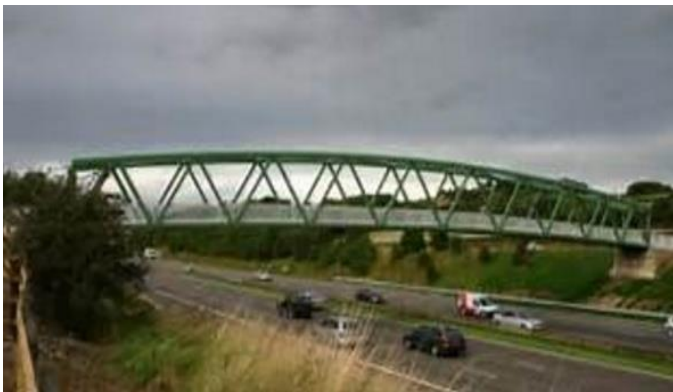
Fig-2: Vierendeel Truss bridge
