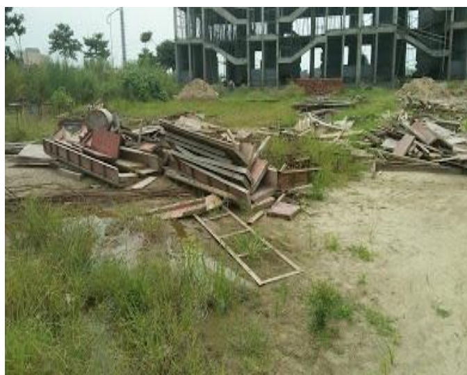
Fig.-3 Shuttering getting spoiled
