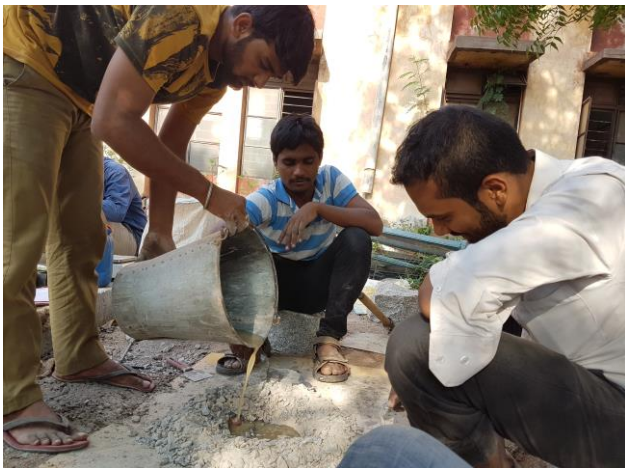
Figure - 1.0 Casting of Geopolymer Concrete.
