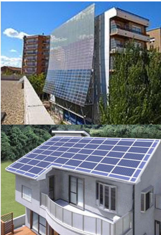
Fig-7: Photovoltaic wall, BIPV
