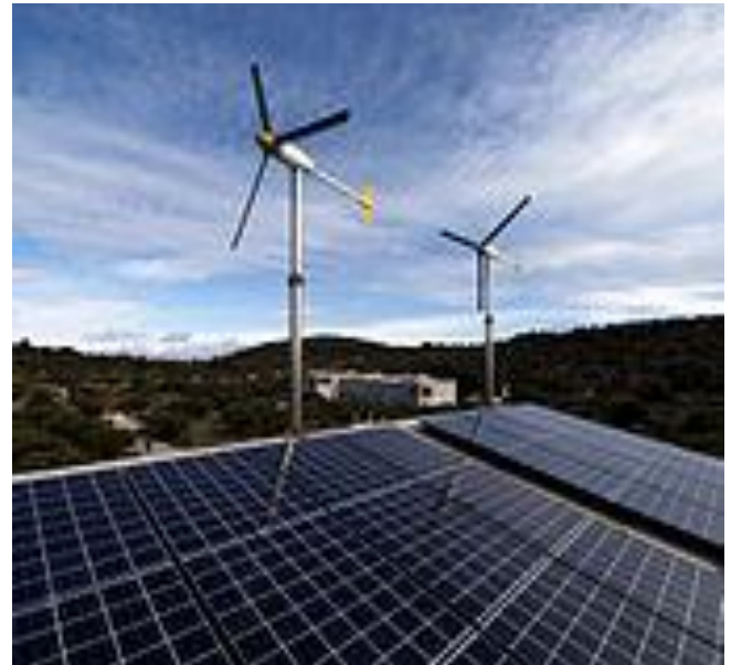
Fig-6: Solar-Wind hybrid systems
